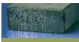
S15 ■ Eroded brush face
